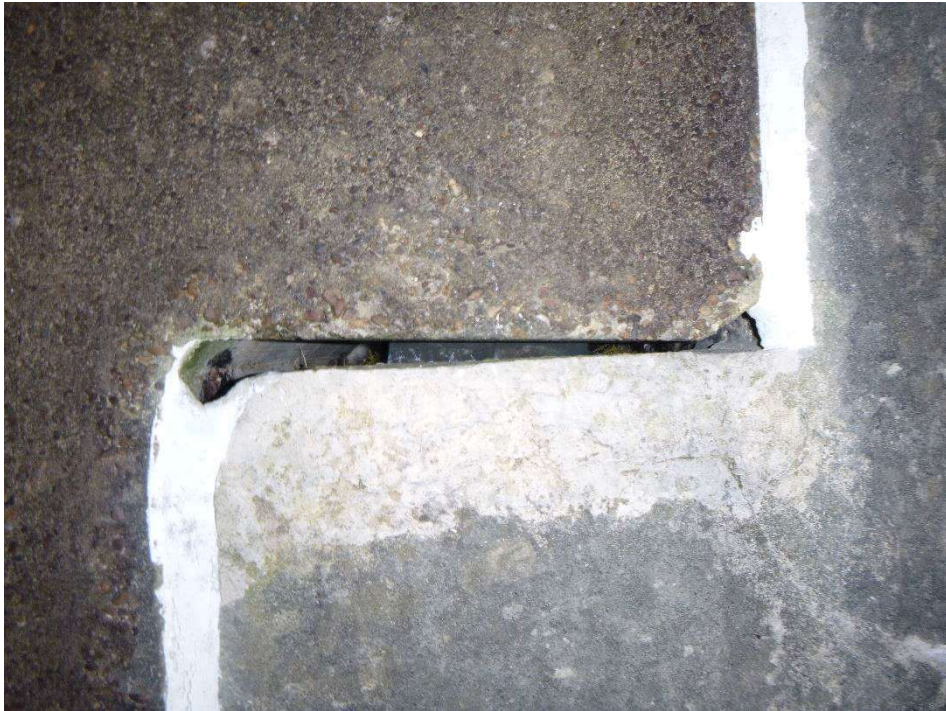
Photograph 13 - East joint south face
