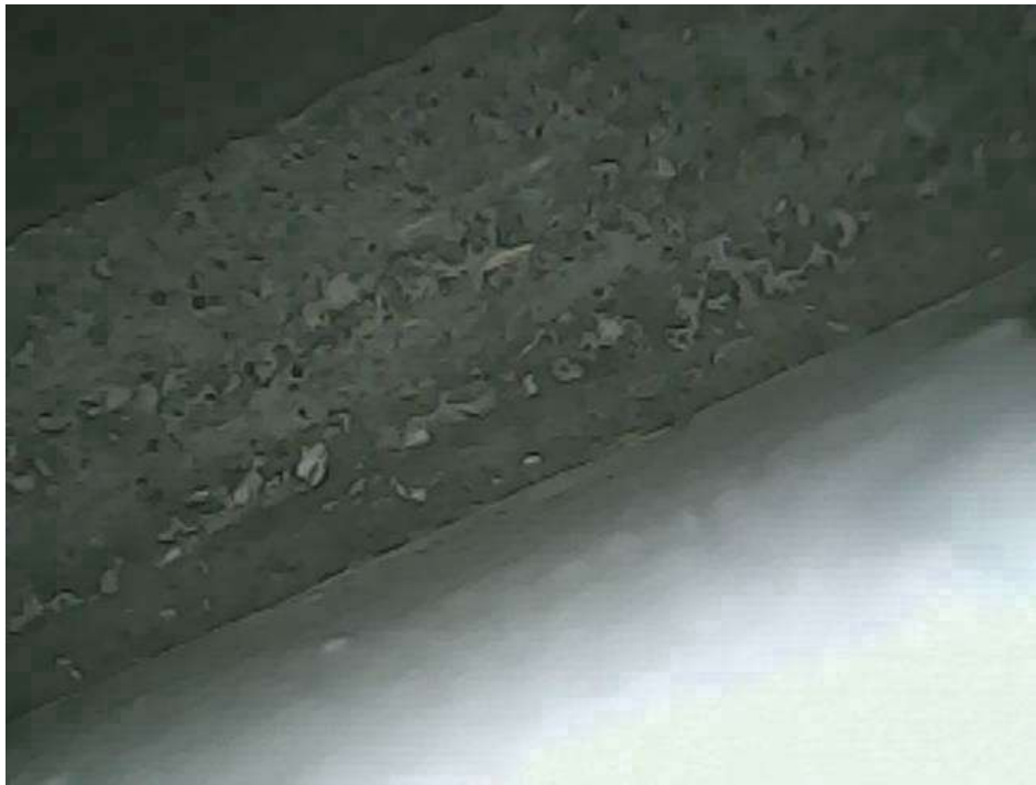
Photograph 30 - Soffit of upper nib, south side.
