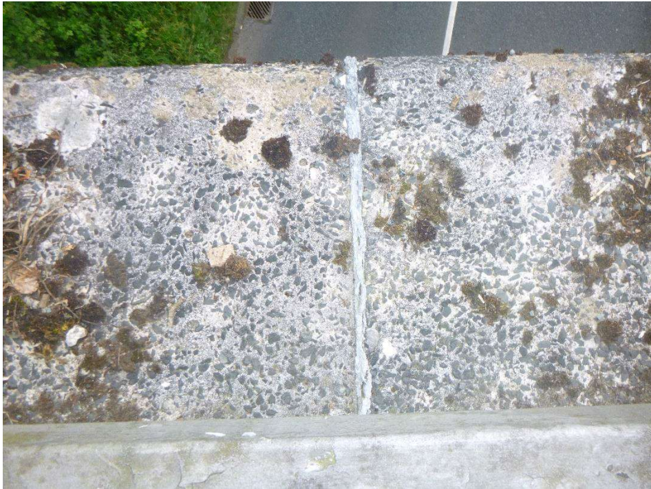
Photograph 27 - West expansion joint, North upstand.
