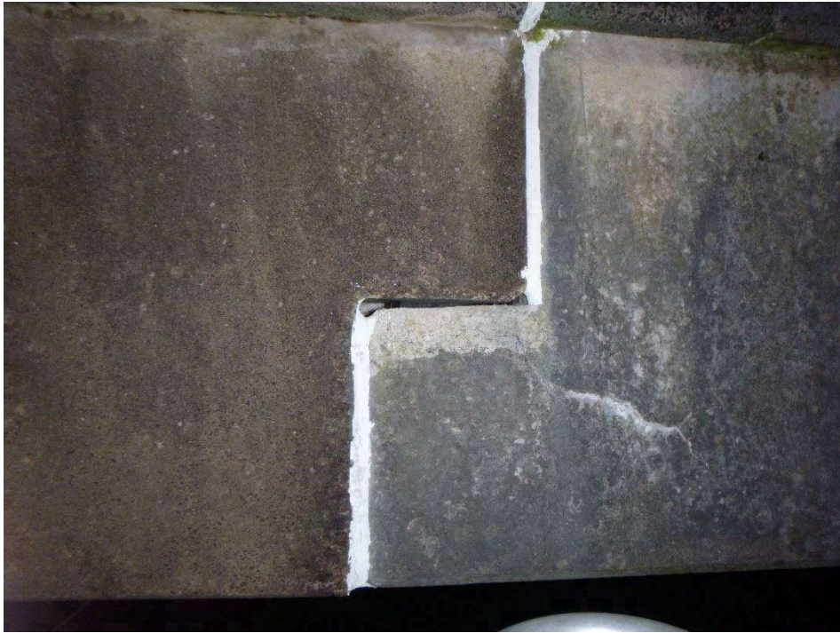
Photograph 9 - East joint south face
