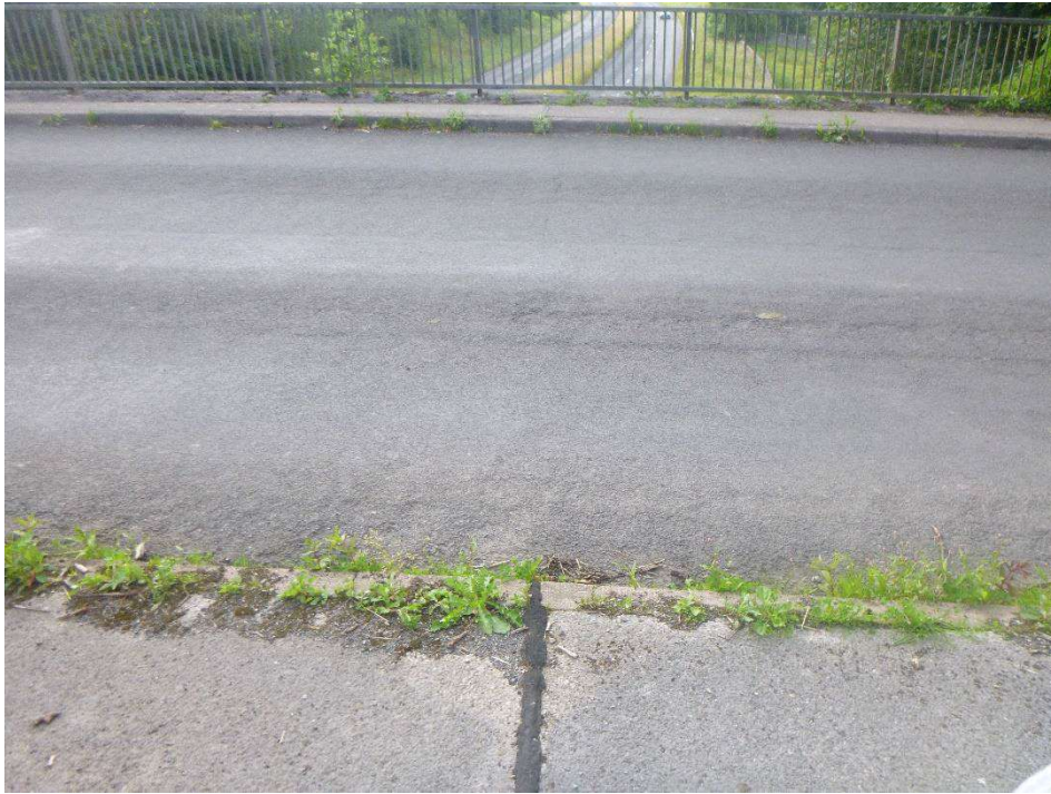
Photograph 5 - East half joint looking north
