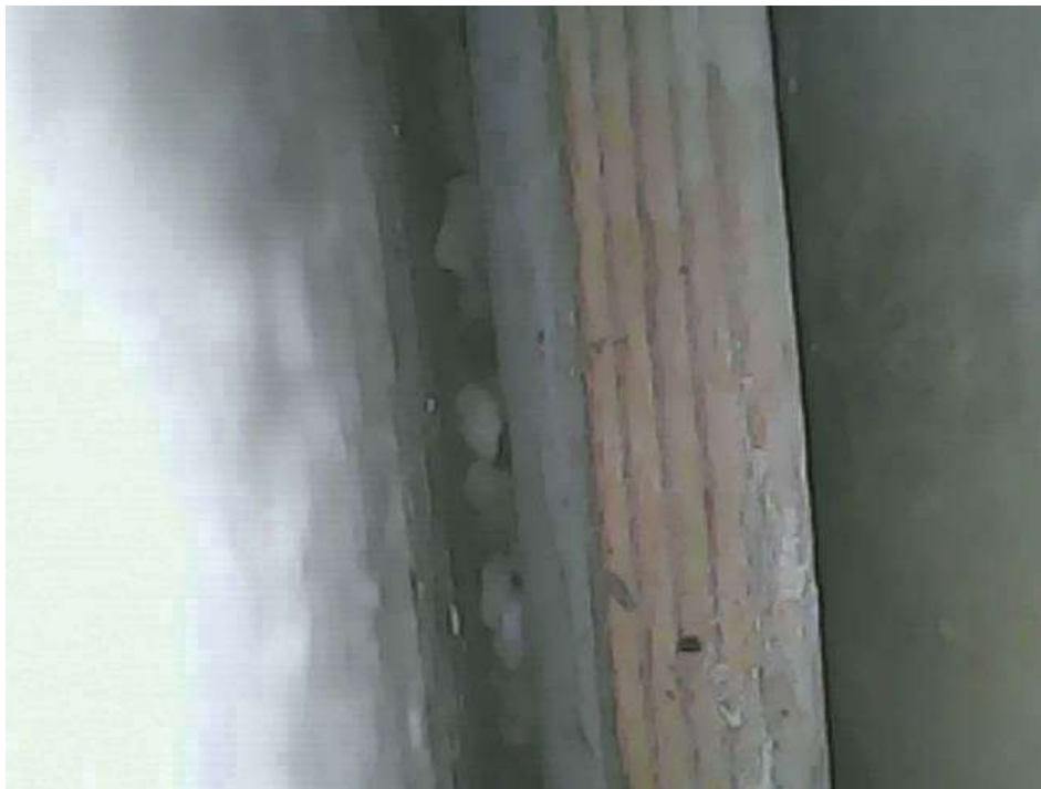
Photograph 12 - East half joint, formwork within joint
