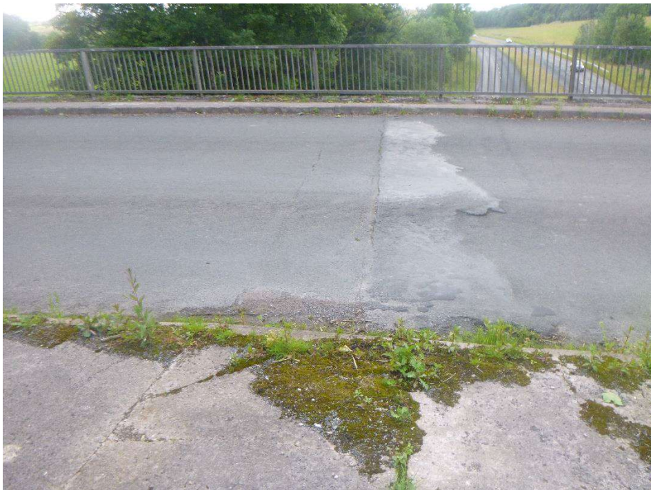
Photograph 24 - West Half joint looking north
