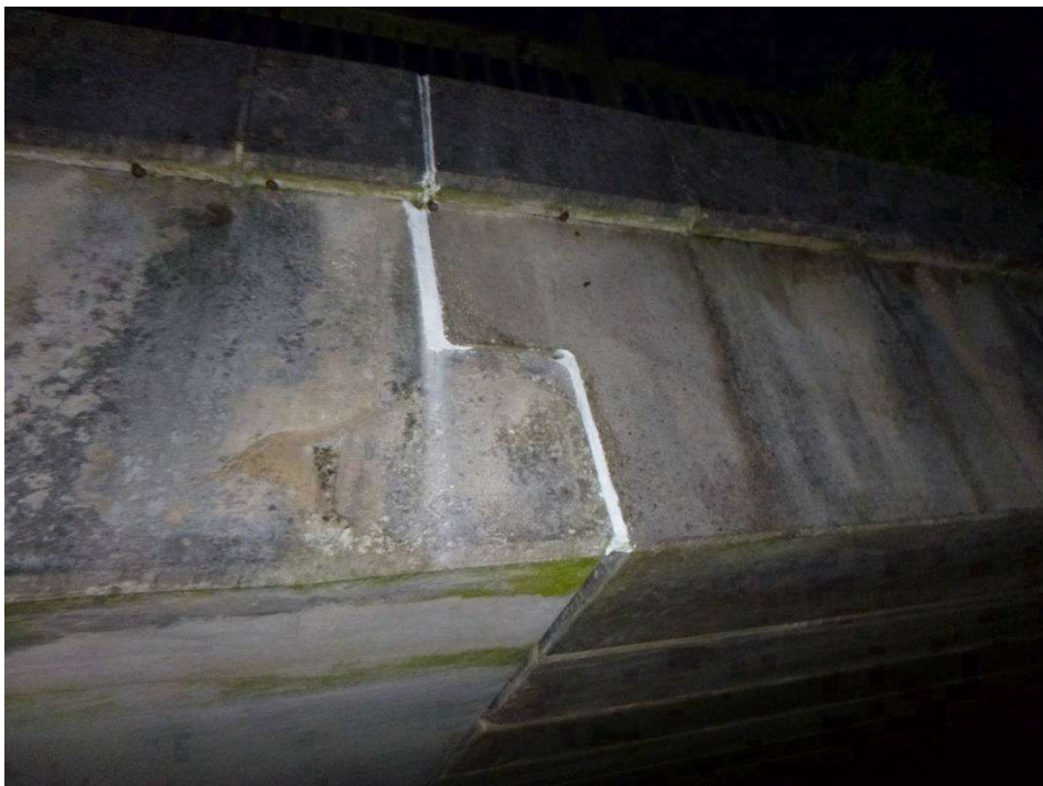
Photograph 10 - East joint north face
