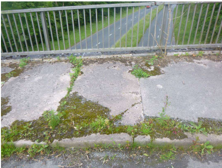
Photograph 26 - West half joint south verge
