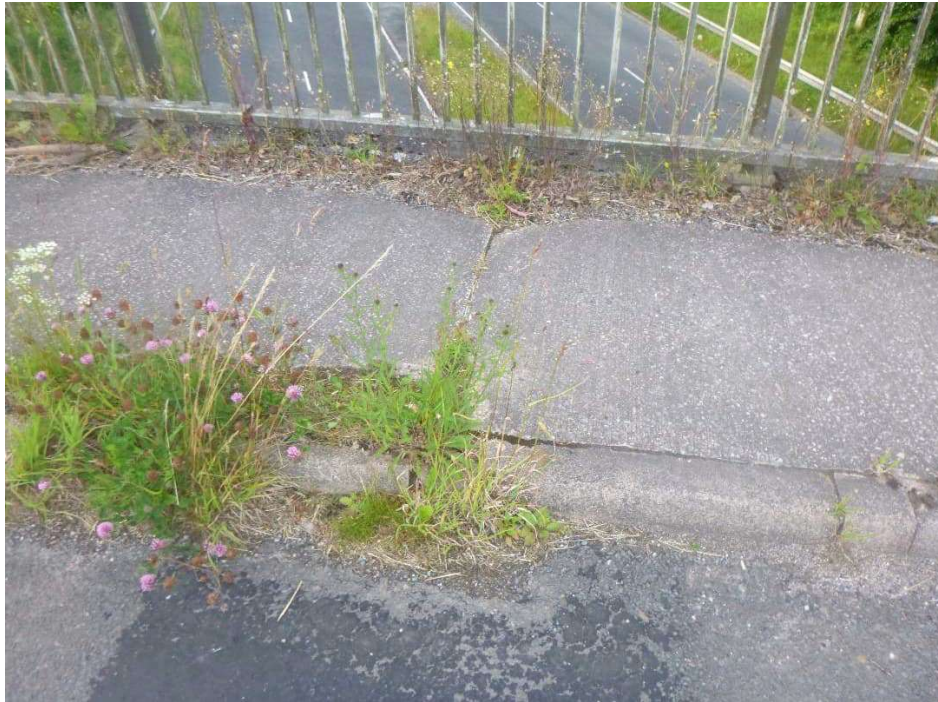
Photograph 29 - North verge west half joint
