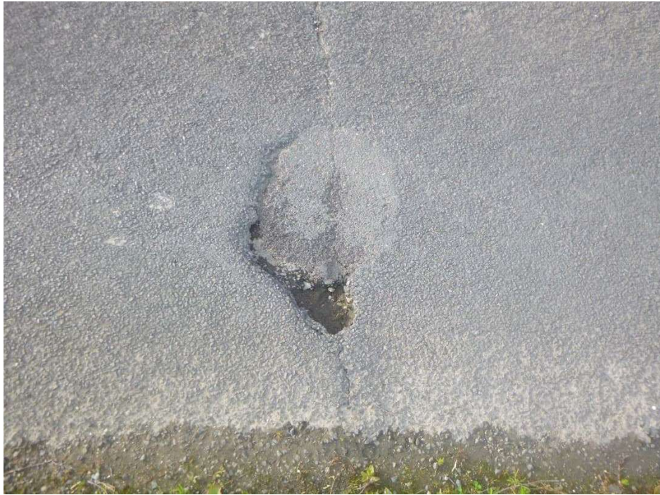
Photograph 7 - Potholing close up on east half joint
