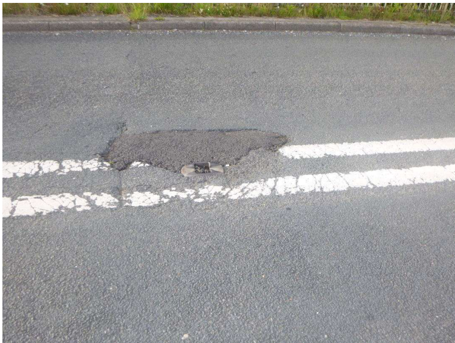
Photograph 8 - Potholing to centreline of carriageway above east half joint
