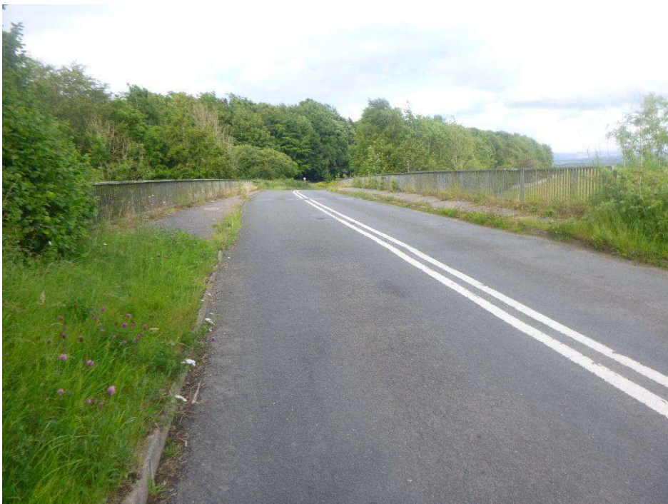
Photograph 2 - View on underbarrow road looking east
