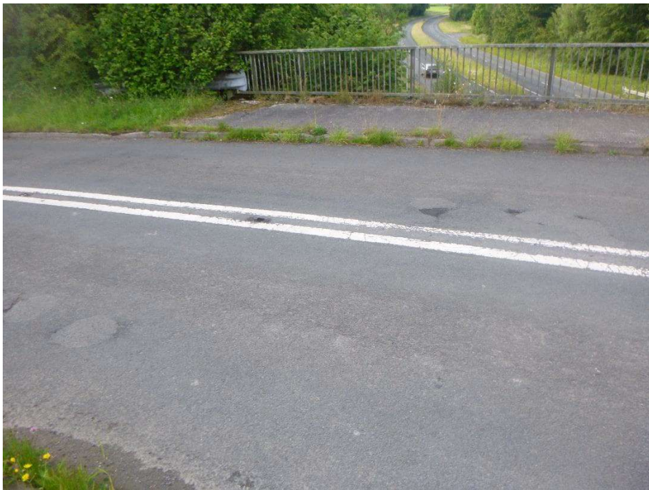
Photograph 32 - Potholing at west end
