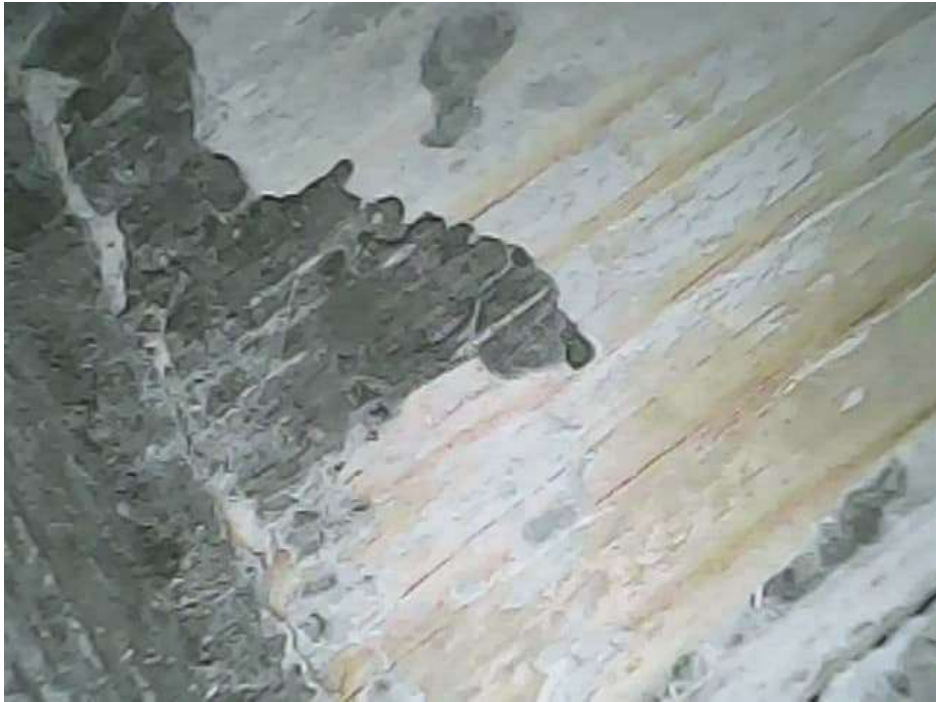
Photograph 11 - Timber formwork left in place between southern beams
