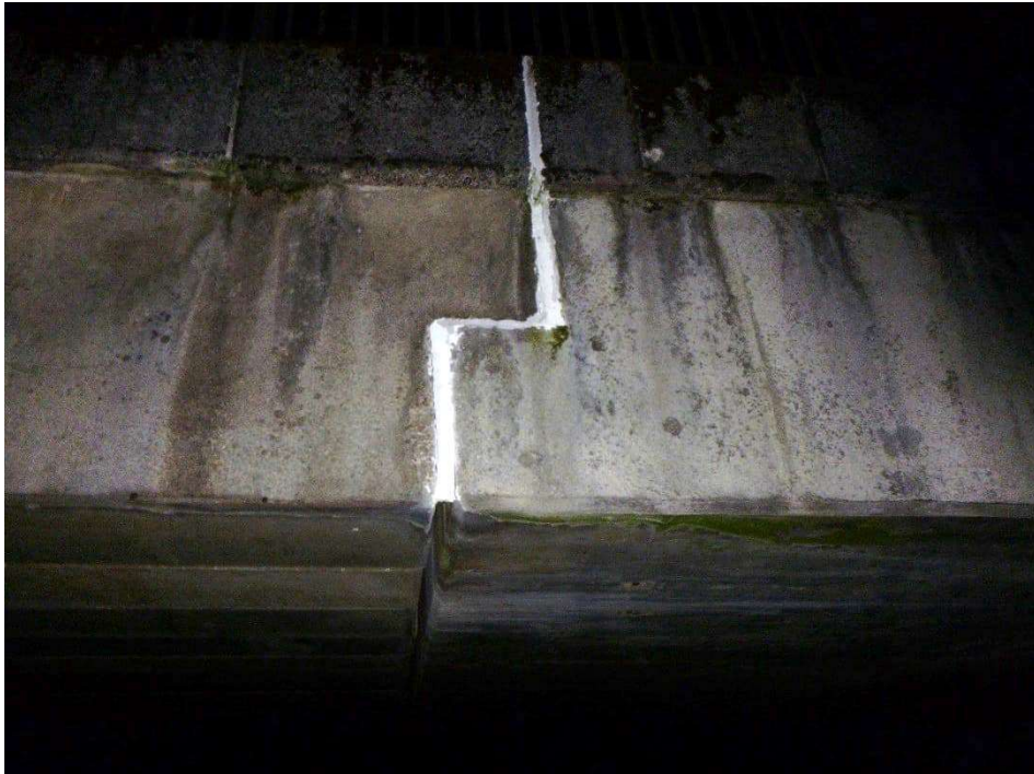
Photograph 35 – North-west half joint
