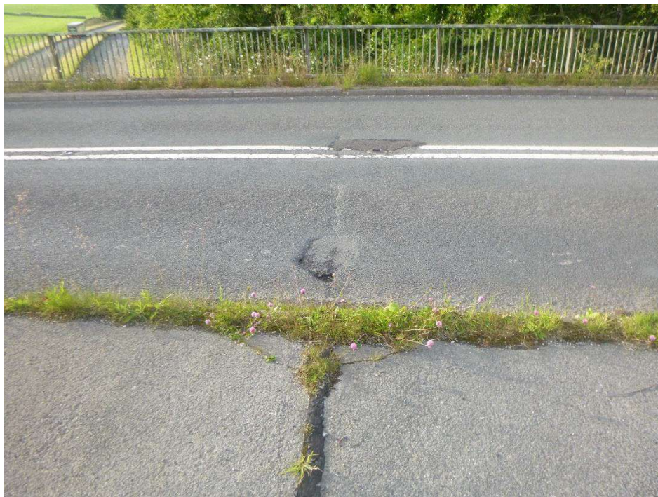
Photograph 6 - View north on east half joint
