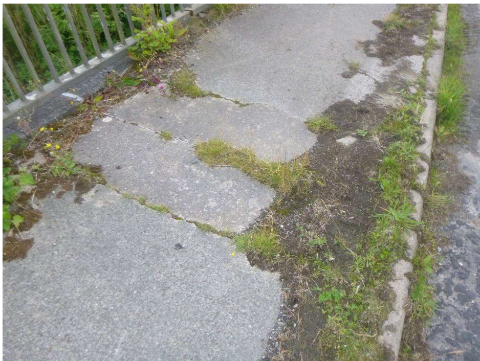
Photograph 30 - South verge west half joint
