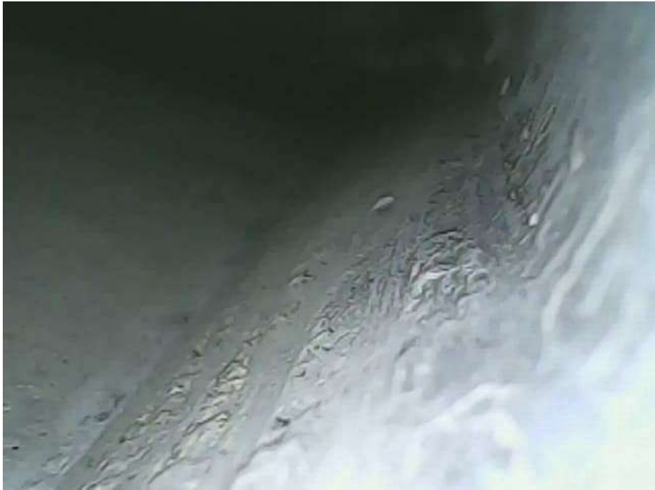
Photograph 39 - Lower nib in good condition
